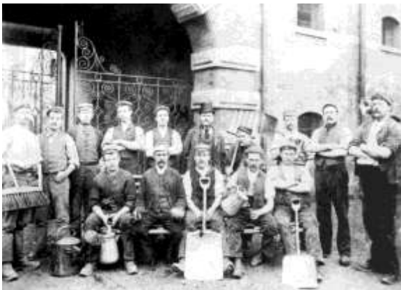
Above Left: Workers at Stones' Malt Kilns in 1905
